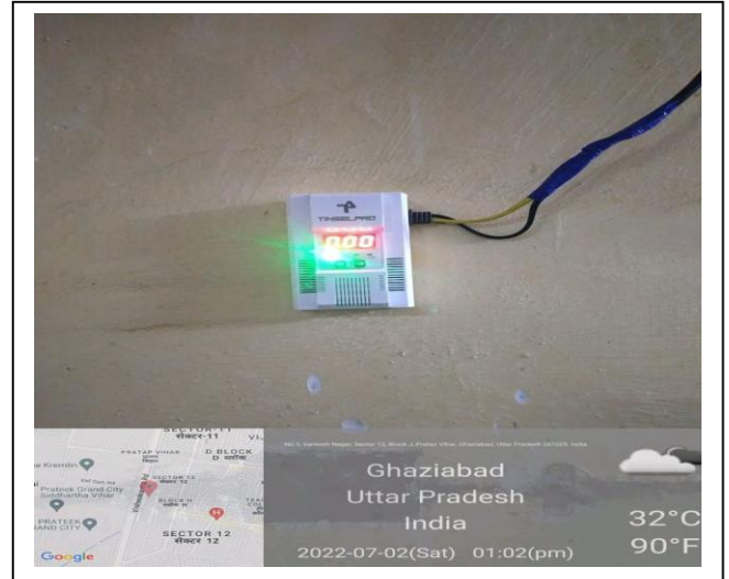
Gas Leakage Sensor in Canteen
