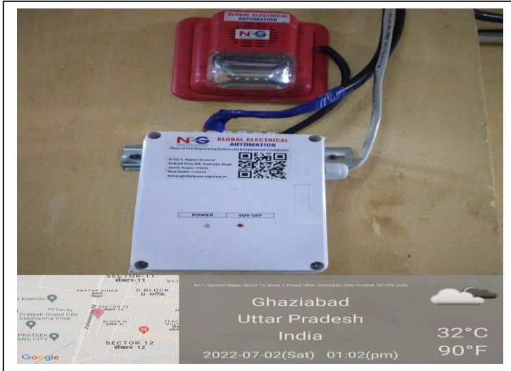
Gas Leakage Sensor in Canteen
